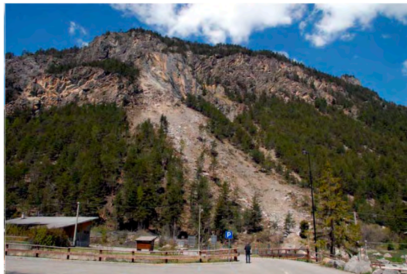
Figure 3. View of the examined rock slope [18].
