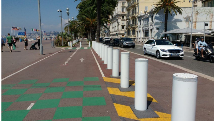
Figure 1. Example of vehicle security barriers (VSB) commonly used in an urban environment
