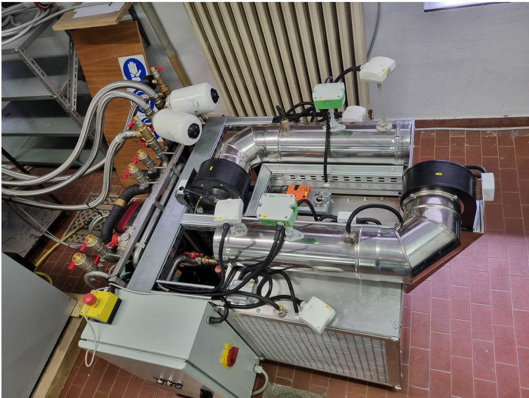
Fig. B.7 Adsorption Unit. Real Prototype
