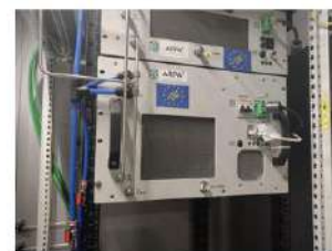
Figure 2 Installed electrolyser at ZEM module
