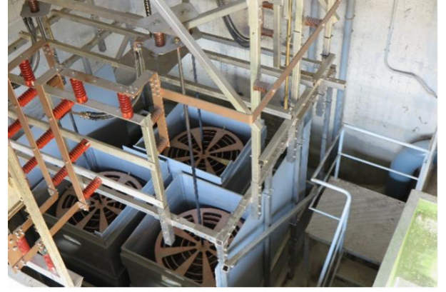
Fig. 3: New design of the power dissipation system.
