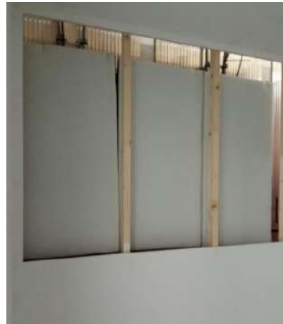
Fig. 6 – Detail of the suspended sound-absorbing panels layered between the wooden structure and beyond the acoustic-transparent membrane
