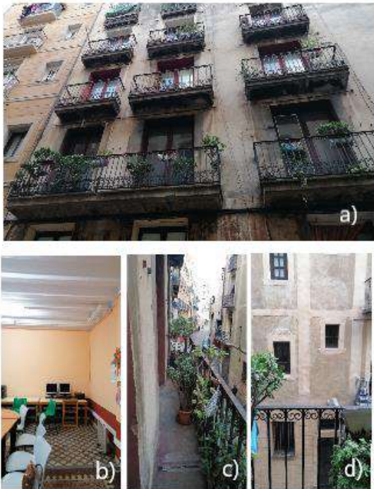
Fig. 7 – The real case study, a classroom in the Raval neighbourhood in Barcelona: a) façade, b) interior with furniture, c) view from the balcony, and d) view of the opposite building
