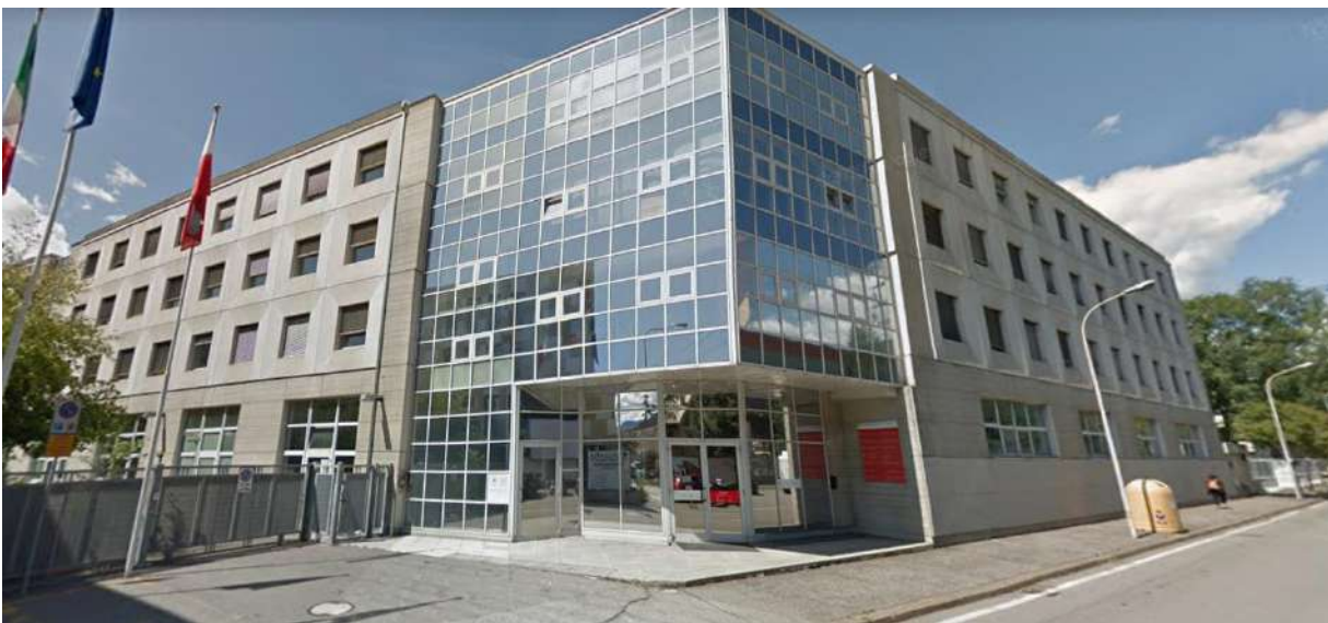
Fig. 1 – Case study building located in Bolzano, Italy
