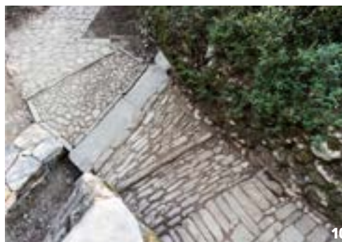
5-7. Working on the kalderimi , the arch and the wall during the first Boulouki workshop. Photo credit: G. Dimitrakopoulos. Source: Boulouki Archive.
