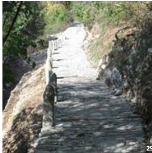
28-29. Before and after the kalderimi reconstruction, and the placement of the upright stones called arkades . Photo credit: G. Koutropoulos, P. Radin and G. Zoilis. Source: Boulouki Archive.
