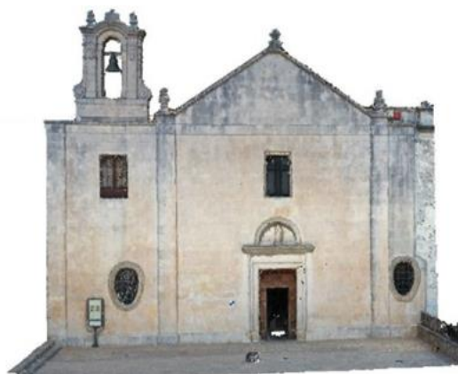
Fig. 3. Point cloud of the external structure generated by photogrammetric survey from UAV.
