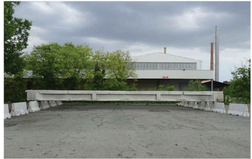
Figure 8. Beams placed sequentially on New Jersey supporting members in the testing site.
