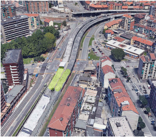
Figure 1. Aerial view of the Corso Grosseto viaduct.
