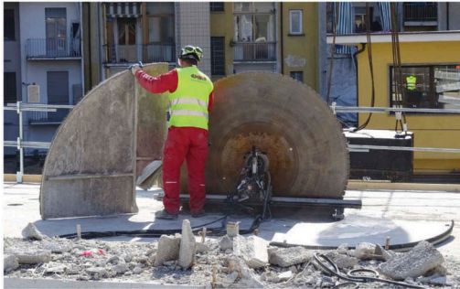
Figure 5. Cutting the beams of the bridge deck.
