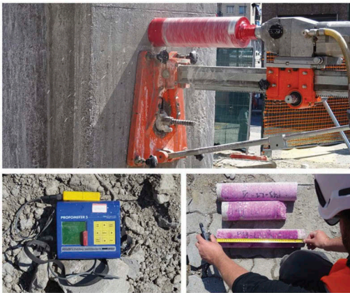
Figure 10. Concrete split coring and carbonation tests.
