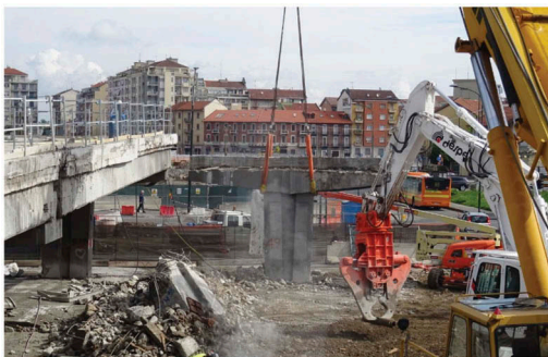
Figure 6. Lifting of a pier cap.
