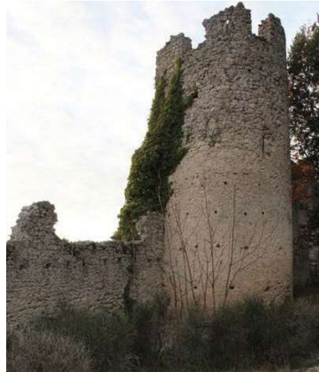
Fig. 13. Central tower with circular holes (2021).
