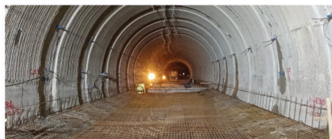
Figure 13. Invert arch reinforcement works for the Bellosguardo tunnel (courtesy of Lapo Baccolini)
