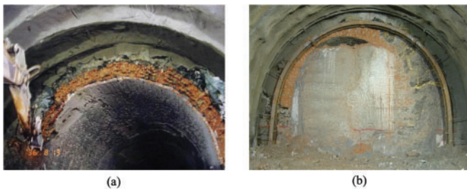
Figure 19. (a) Berry Street tunnel enlargement 55 and (b) concrete-filled section of the Grazia Bassa tunnel 61
