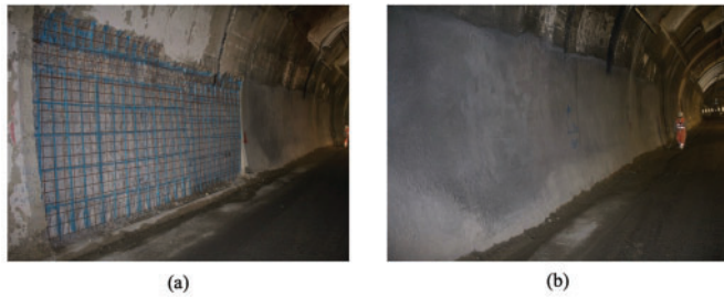
Figure 8. Rebar corrosion protection intervention in the Monte Baldo tunnel: (a) exposed rebars treated with protective coating and (b) concrete cover reconstruction
