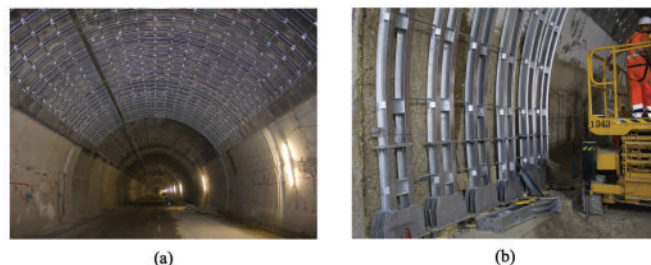
Figure 12. Installation of (a) dowelled steel ribs in the Monte Baldo tunnel and (b) ground-footed steel ribs in the Pozzolatico tunnel
