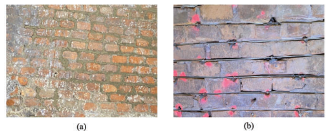
Figure 10. Bed joint remake of a motorway masonry tunnel in Italy through (a) high-performance mortar and (b) steel tendons (courtesy of Lapo Baccolini)
