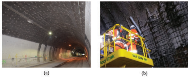
Figure 5. Installation of (a) protective steel nets in the Citerna tunnel and (b) Ram-Arch ® system in the Whiteball tunnel 38
