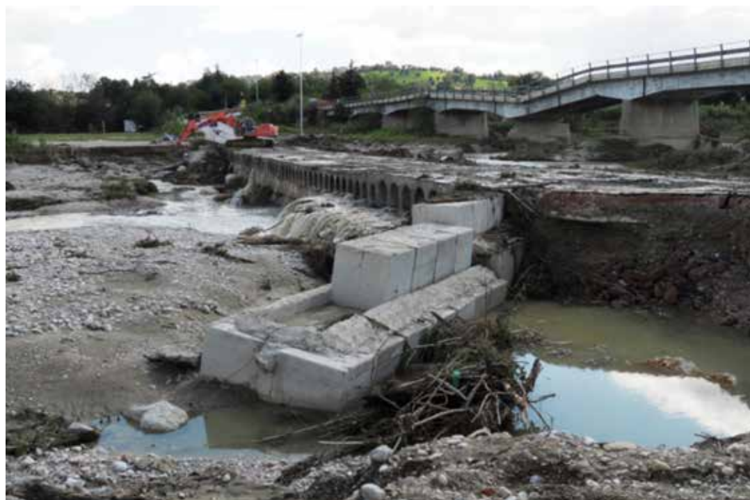
Fig. 5: Degraded landscapes. Hydrogeological instabilities caused by the poor interaction of nature and human intervention: the Fiastra River near Sforzacosta (MC)
