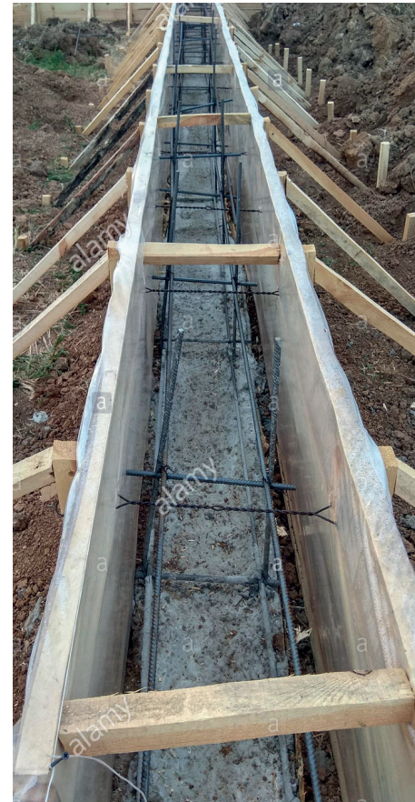
Cassero in legno da https://www.alamy.it/cassero-in-legno-cemento-fondazione-striscio-per-un-cottage-2018-image219021678.html
