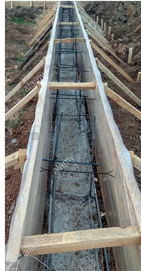
Cassero in legno da https://www.alamy.it/cassero-in-legno-cemento-fondazione-striscio-per-un-cottage-2018-image219021678.html
