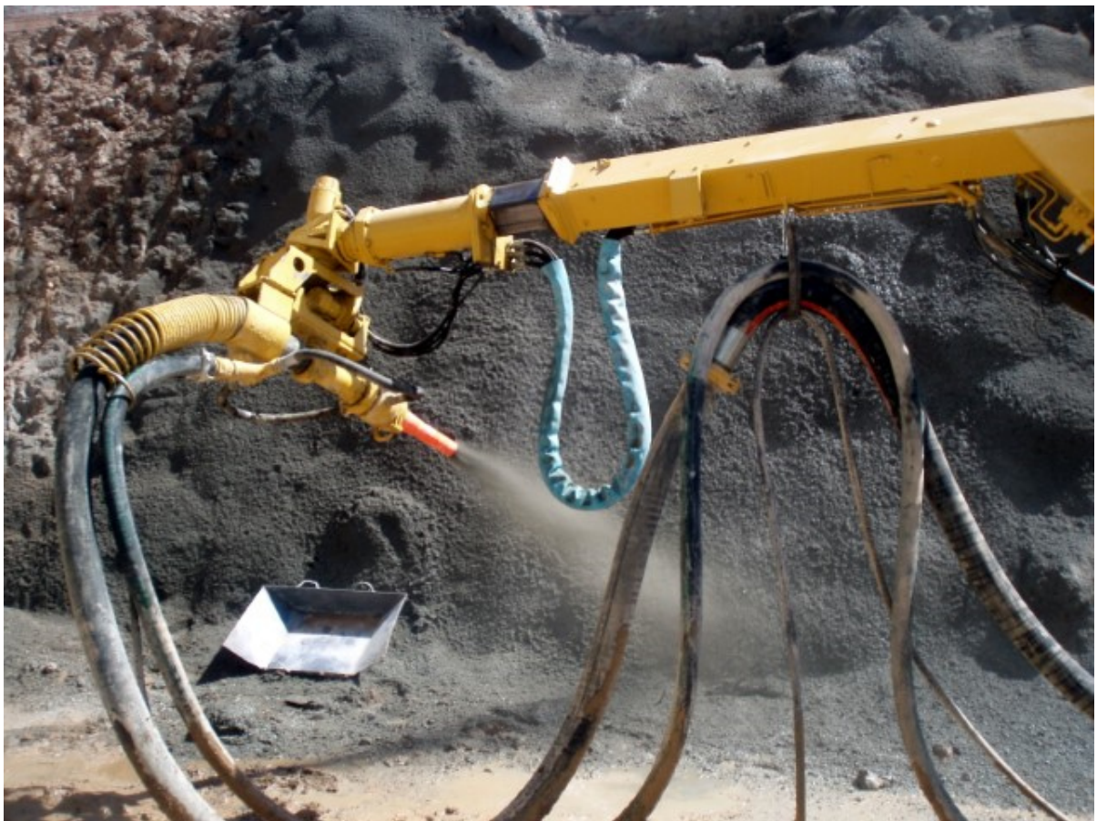
77 Fig. 1 Application of shotcrete
