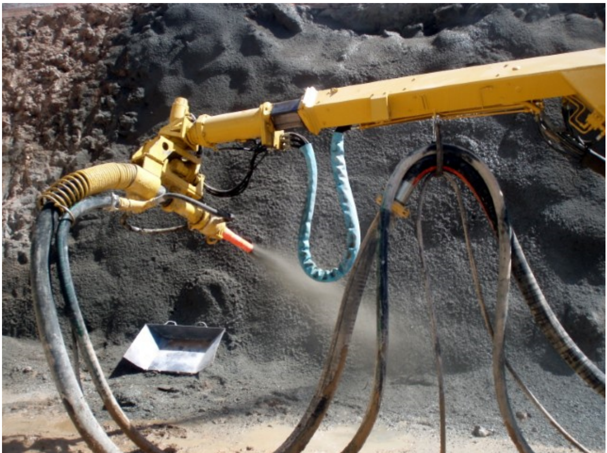
Fig. 1 Application of shotcrete
