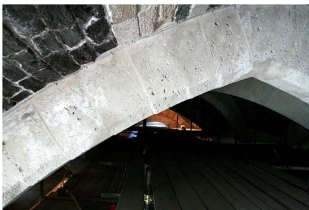
Figure 10 The classical sliding mechanism (as a consequence of the springing displacement) surveyed on the voussoirs of the pointed arches rising from the trilobate columns.
