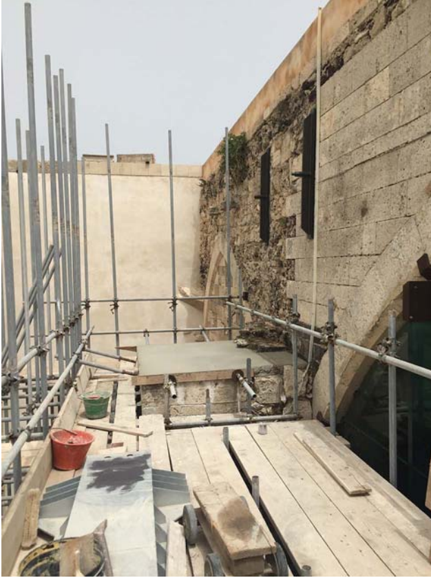
Figure 26 Picture of the anchor plates to sustain the façade.
