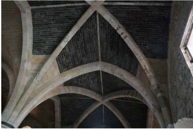
Figure 3 Restoration works on the cross vaults of the Salone carried out after the 1693 earthquake, involving the replacement of the original web stones by lighter lava stones.
