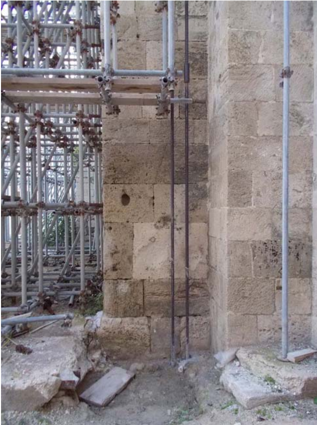
Figure 29 Side view of the right buttress with the tendons and the anchor bars aligned and bounded by static couplers.
