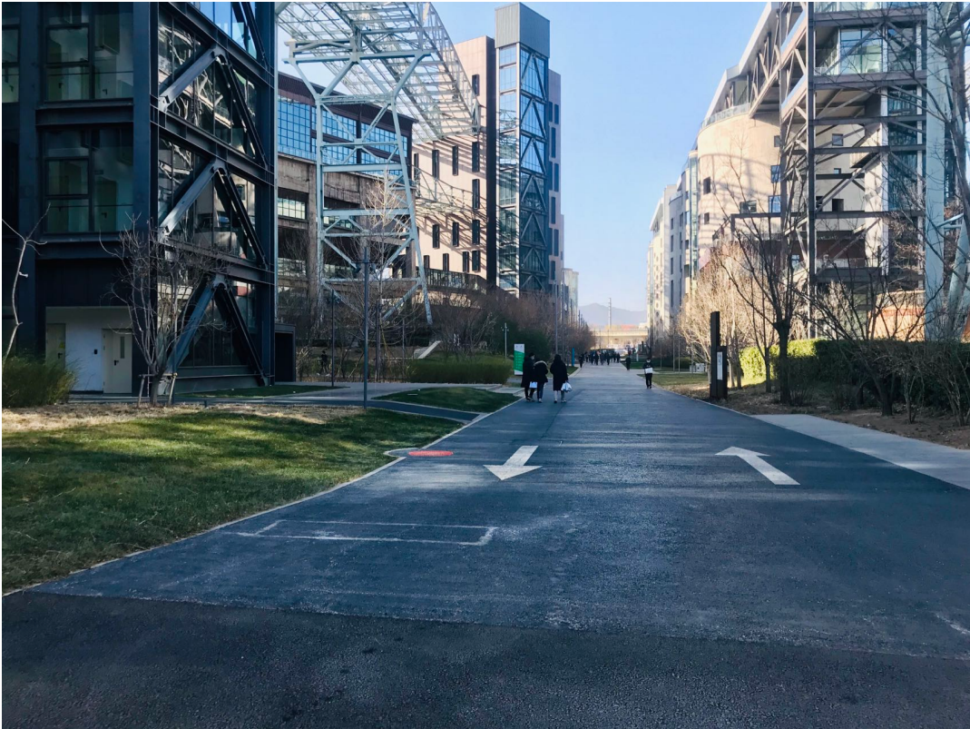
Figure 4.12 BOCOG headquarter in Shougang Industrial Park in ex silos. (Source by the author). In 2019, Big Air platform 30 was inaugurated, with a structure and colors designed to be as light as possible and to resemble a flying ribbon, as a landmark that makes a direct echo to Chinese culture and aesthetics [Figure 4.13 and Figure 4.14].
