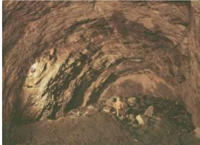
107 108 Figure 1. Primolano tunnel (Italy). High quality of the tunnel contour, half blasthole clearly evident at ribs and crown. 109 Suggested D = 0 . (Courtesy Italesplosivi) 110
