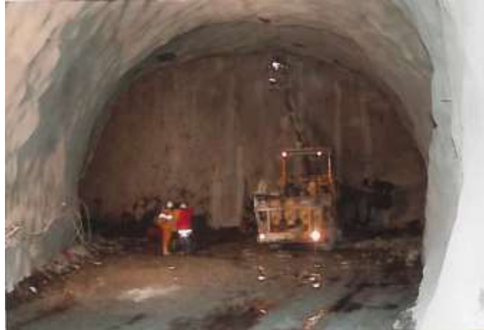
111 112 Figure 2. Irregular tunnel contour after D&B; shotcrete for the first phase support is smoothing asperities and over 113 excavation, but nominal profile is not obtained yet. Suggested D = 0.7 . (Anonymous)
