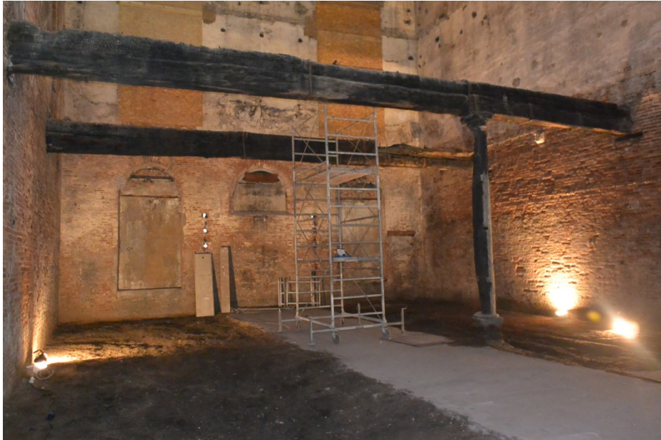
Fig. 7 Interior view of the Sala d'Armi "E", composite beams and wooden column (Photo D. Ferrante, 2019)
