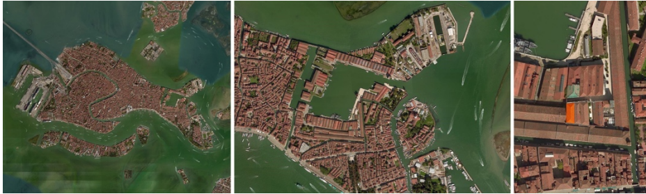
Fig. 1 Aerial view of the city of Venice (a), the Arsenale complex (b) and the Sale di'Armi (Room E highlighted in orange) (c)
