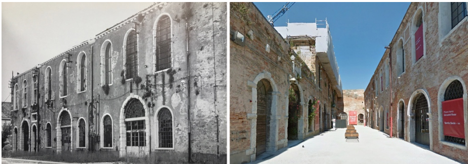
Fig. 4 View of the Sala d'Armi South, 1980's (left) (from U. Pizzarello, V. Fontana, 1983); Sala d'Armi North and South during the recent restoration.
