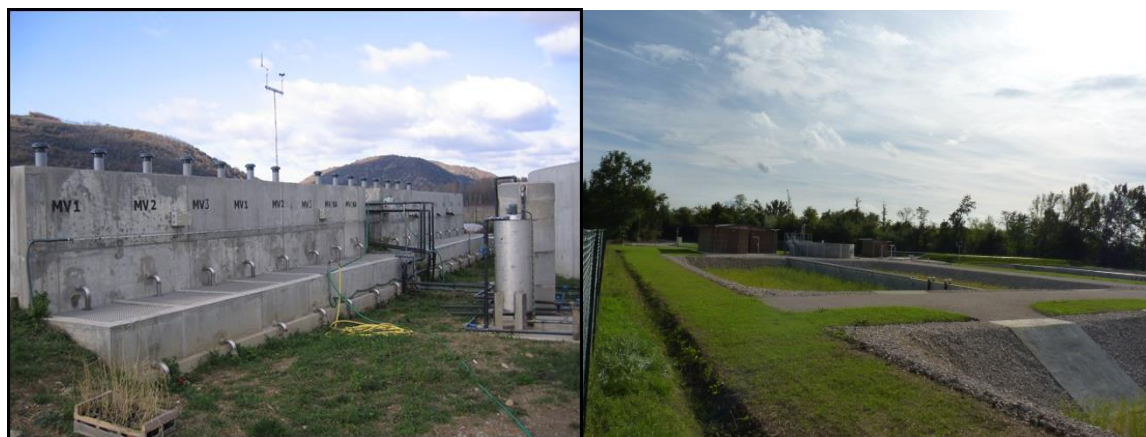
Figure 1. Pilot and full scale device for septage treatment.
