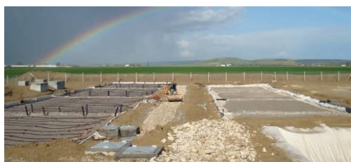
Chorefech (Tunisia) CW WWTP under construction in 2008
