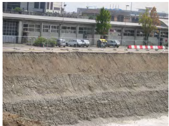
Fig. 17 - An approximately 15 m deep recent building excavation within Turin (Giordano Bruno Street, G in Fig. 14) shows the sequence formed by gravelly and sandy outwash sediments, supplied by the Dora Riparia River during the Upper Pleistocene.
