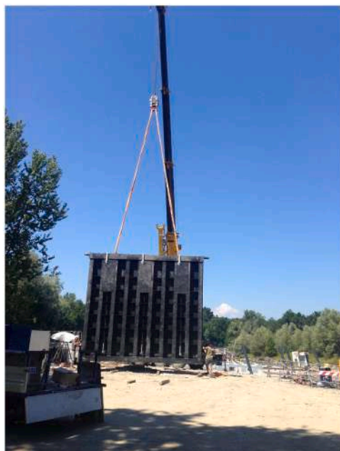
(a) Transport and unlift by crane
