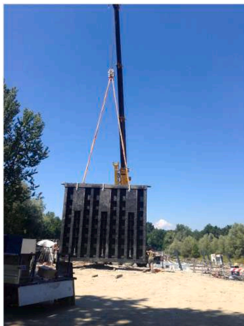
(a) Transport and unlift by crane
