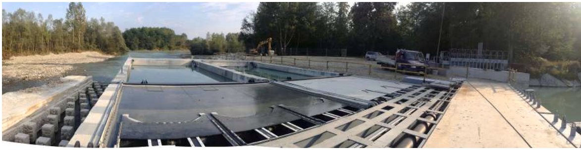
Fig. 15. VLHT installation in the canal, Mazzè, Italy.
