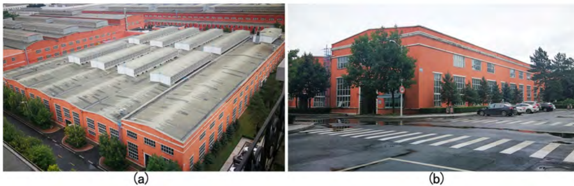
Figure 24. The Harbin Boiler Factory: (a) the roof and the external design of Welding Workshop and (b) the facade of Welding Workshop.
