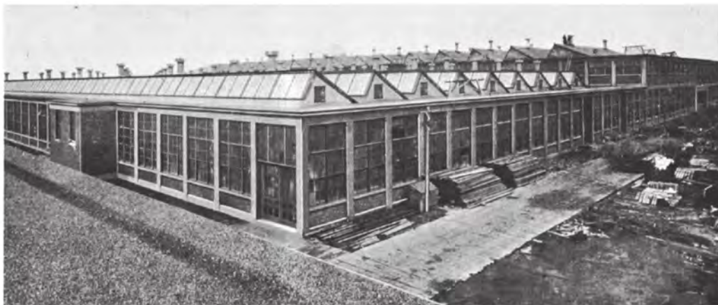
Figure 6. The continuous zigzag roof windows of the Pierce Plant workshop. (Source: [8]).
