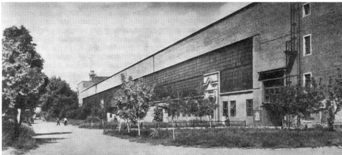
Figure 16. The workshop of the Kramatorsk Plant. (Source: [45]).
