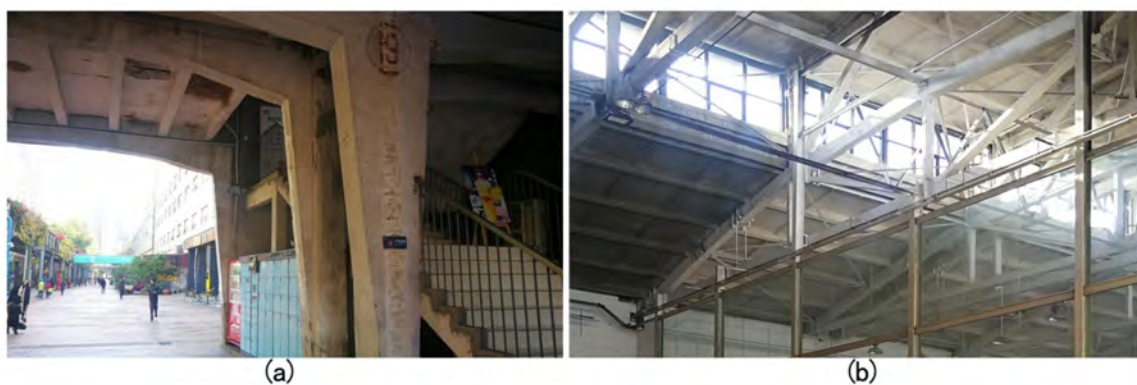
Figure 27. The Chengdu Hongguang Electronic Transistor Factory: (a) the reinforced concrete structure of Assembly Workshop (b) the steel frame roof truss of Testing Workshop.
