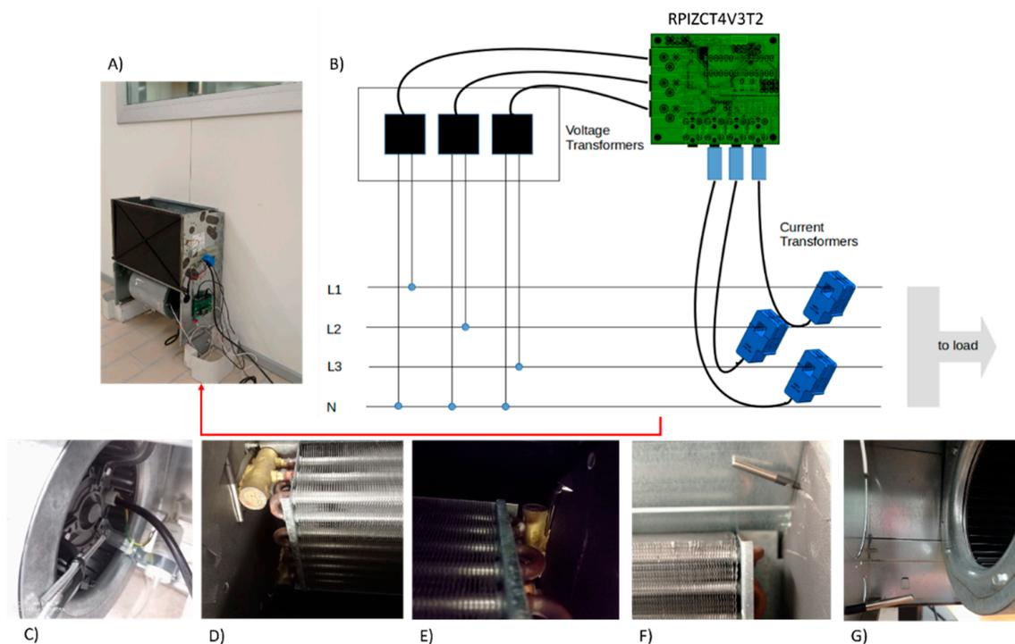
**Figure 8.** Sensors allocation on the FC components: (A) FC equipped with sensors; (B) Connecting and measuring diagram of the current and voltage of the FC motor; (C) T5 sensor connected to the motor case; (D) T2 return pipe sensor; (E) T1 delivery pipe sensor; (F) T3 air intake sensor; (G) T4 air outlet sensor.
