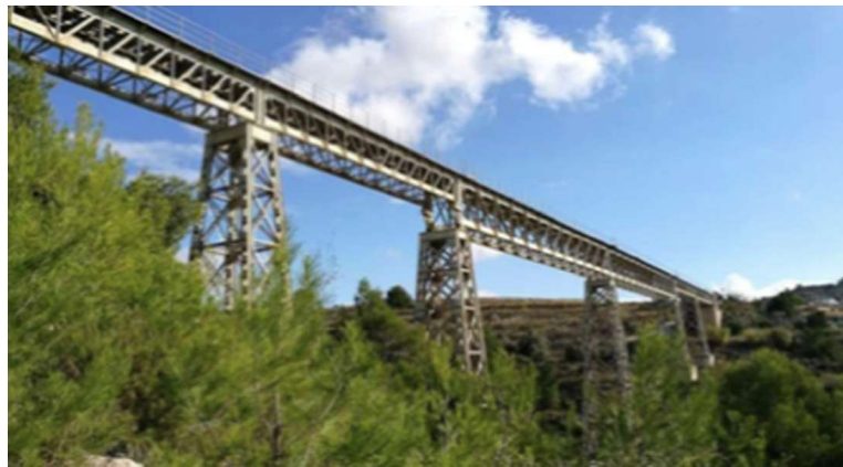
Fig. 1. Quisi (railway) steel truss bridge-Benissa
