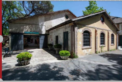
CARPENTERS' WORKSHOP IS CONVERTED INTO EXHIBITION CENTER DEDICATED FOR THE SUMERBANK INDUSTRIAL CULTURE IN 2021; KUNDURA ARCHIVE
