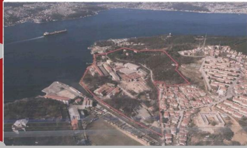
PROJECT AREA UNDER THE SUBJECT OF PRIVATIZATION, KÜNDURA ARCHIVE
