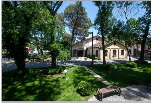
CARPENTERS' WORKSHOP IS CONVERTED INTO EXHIBITION CENTER DEDICATED FOR THE SUMERBANK INDUSTRIAL CULTURE IN 2021; KUNDURA ARCHIVE
