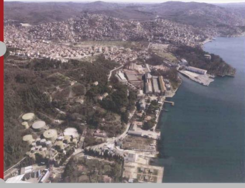
2011 AERIAL PHOTO TO SEE THE PHYSICAL LAYOUT OF THE CAMPUS, KÜNDURA ARCHIVE
