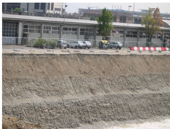
Fig. 17 - An approximately 15 m deep recent building excavation within Turin (Giordano Bruno Street, G in Fig. 14) shows the sequence formed by gravelly and sandy outwash sediments, supplied by the Dora Riparia River during the Upper Pleistocene.
