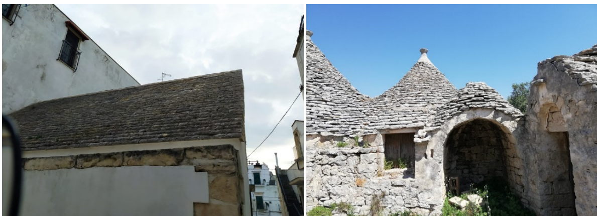
Figure 3: on the left) a modern building with sawn limestones replacing traditional chiancarelle of the roof (cortesy of arch. Intini 2020); on the right) a typical trullo in Itria Valley.
