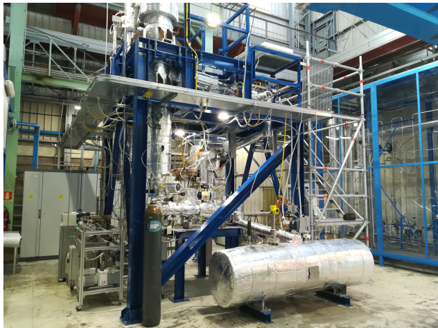
Figure 2: TRIEX-II LiPb facility.
