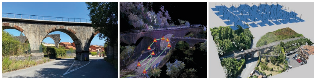
Fig. 1. The result of the survey campaign for a three-arch bridge in the municipality of Mascali (CT). The instruments used are: a NIKON D5300 (photogrammetry), Leica BLK360 (TLS), DJI MAVIC 2 PRO (UAV photogrammetry).
