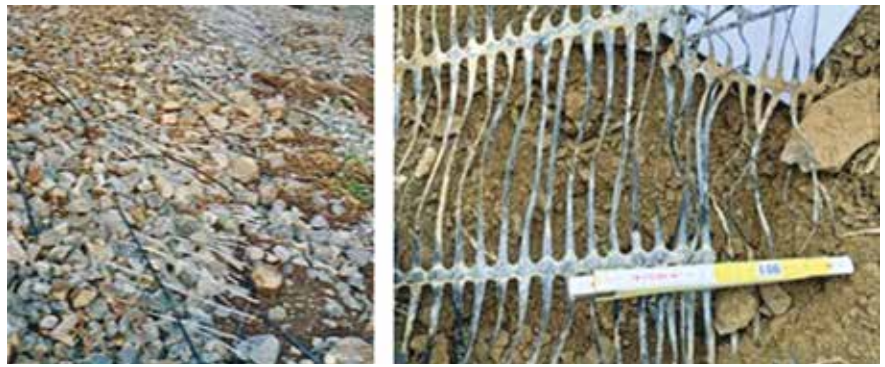
Fig. 2 – Typical tension cracks formed inside the disassembled body of the embankment: on the left woven geogrids elongated in collapsed earth support structure; on the right extruded geogrid elongated after the impact of the block in a protection embankment. Same graphical scale. (credits personal archive C.Oggeri).
