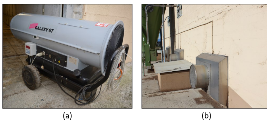
Figure 3.14 – Figure (a) diesel fuel air heater adopted for the supplemental heating; Figure (b) fans for pit ventilation (detail of house B).
