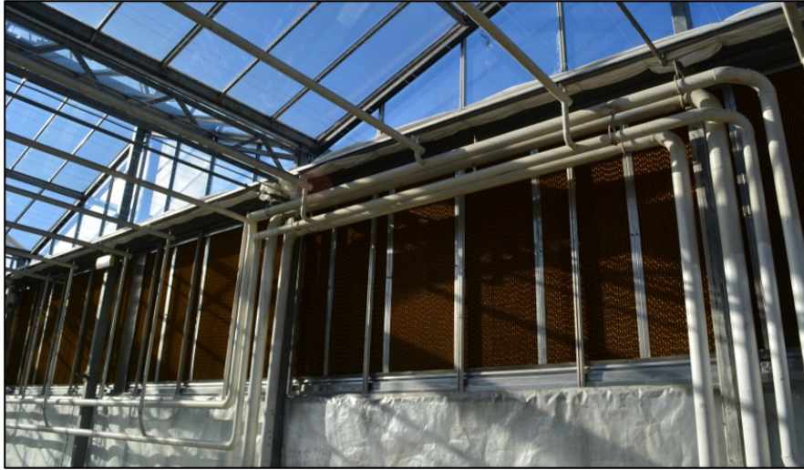
Figure 3.3 - Evaporative pads installed in the monitored greenhouse.
