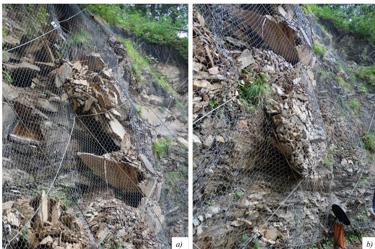
Figure 2. Beneficial effect of the ropes, which prevent failure diffusion near the anchors (a) and provide constraints for the mesh similar to those of standardized laboratory tests of UNI 11437 (b).
