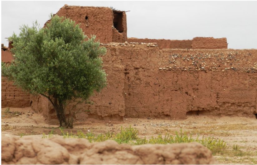
Fig. 1 Adobe rural architecture in Morocco (by M. Mattone, 2015)
