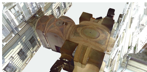
Figure 4. Point cloud of the vaulted system of the Capris di Cigliè palace. The HDR of the cameras attached to the Focus 3D x 130 scanner provides colours close to reality (processing by C. López González).
