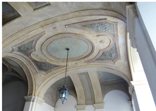
Figure 1. The main banded vault of the atrium of Capris di Cigliè Palace (photo by M. Vitali).
