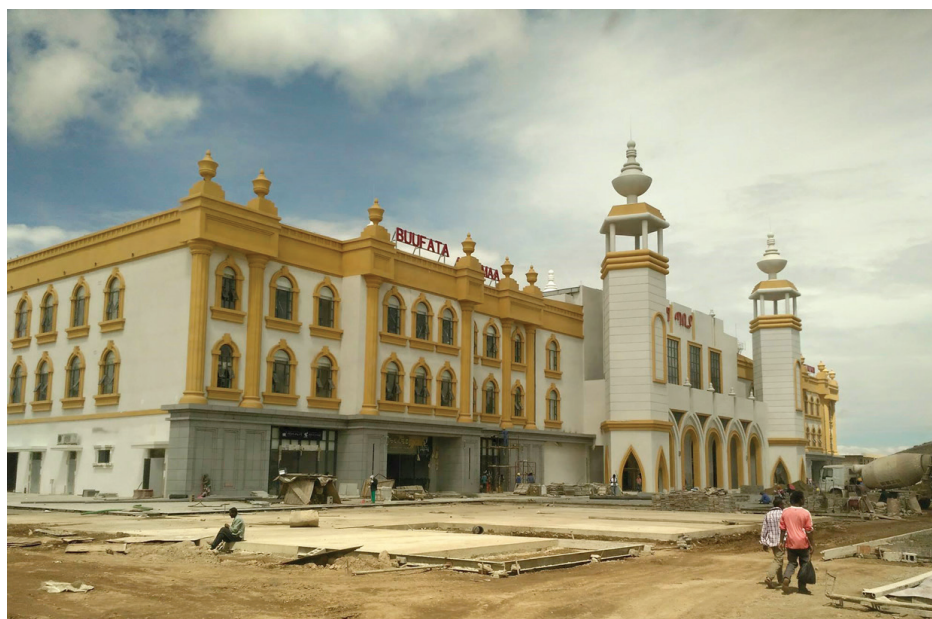
fig. 2.22 - The new Adama train station, photograph, 2017.
