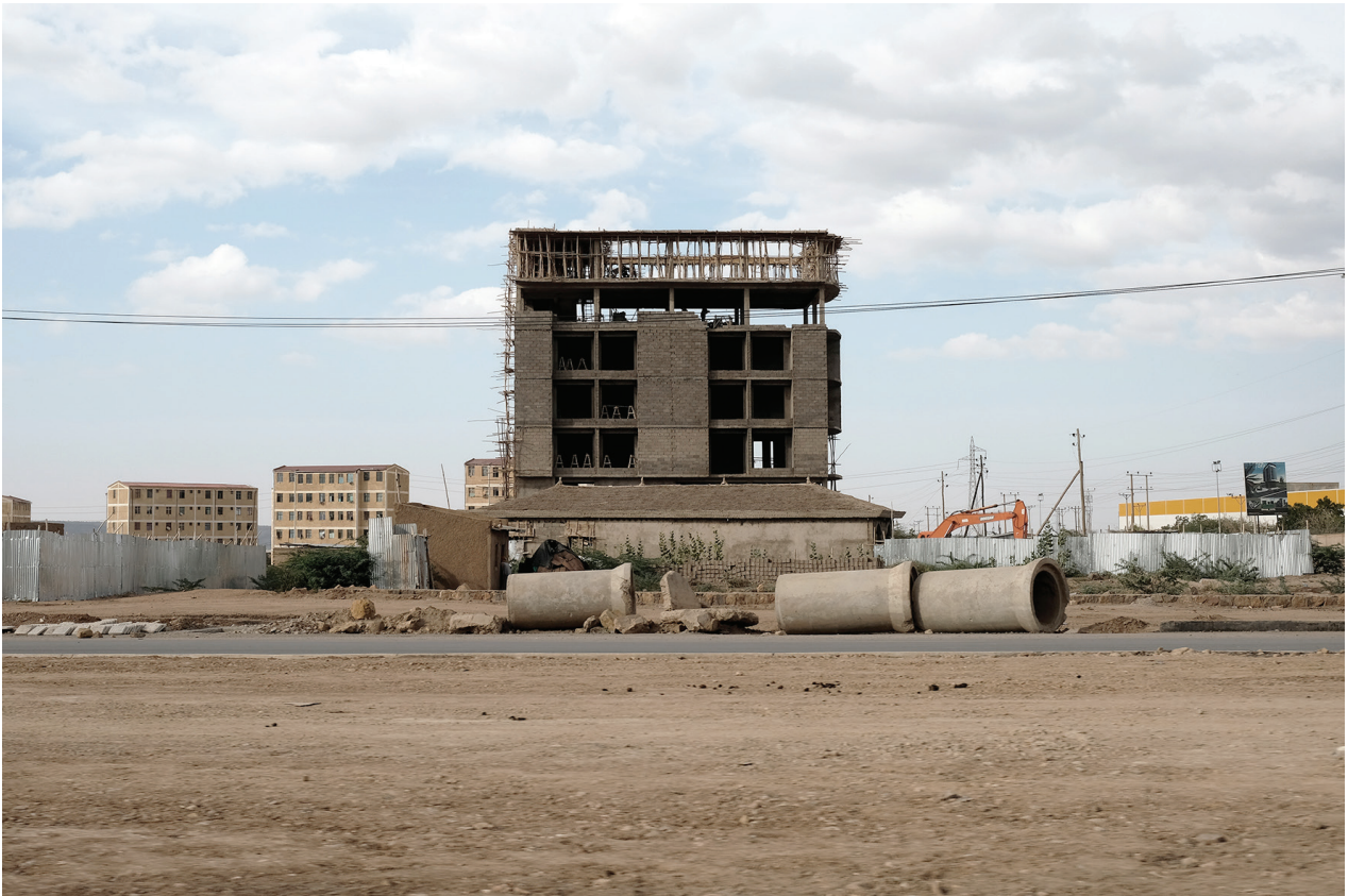
fig. T3.3, fig. T3.4 - Urbanscape along the road connecting the two Dire Dawa stations, photographs, 2019.
