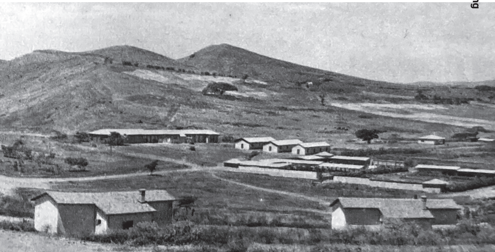
fig. 3.15 - Early construction stage of Bishoftu ONC rural settlement, photograph, 1938.
