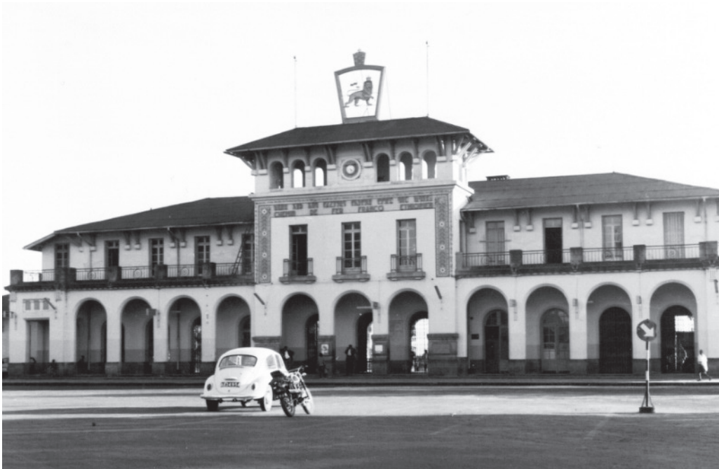
fig. 2.13 - The main facade of the Addis Ababa station, photograph, 1972.
