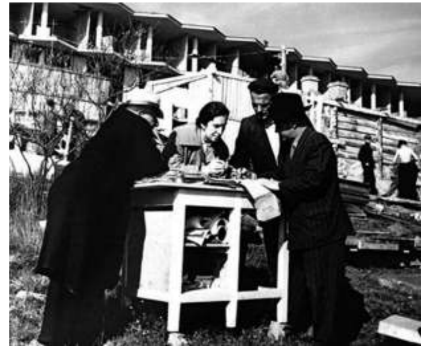
Fig. 1. Natalia Chmutina at the construction site of a hotel in Kyiv, 1962. Source: Olena Maznichenko (ed.), Nataliia Borysivna Chmutina: Zhyttievyi ta tvorchi shliakh arkhitektora (Kyiv, 2012), 143.
