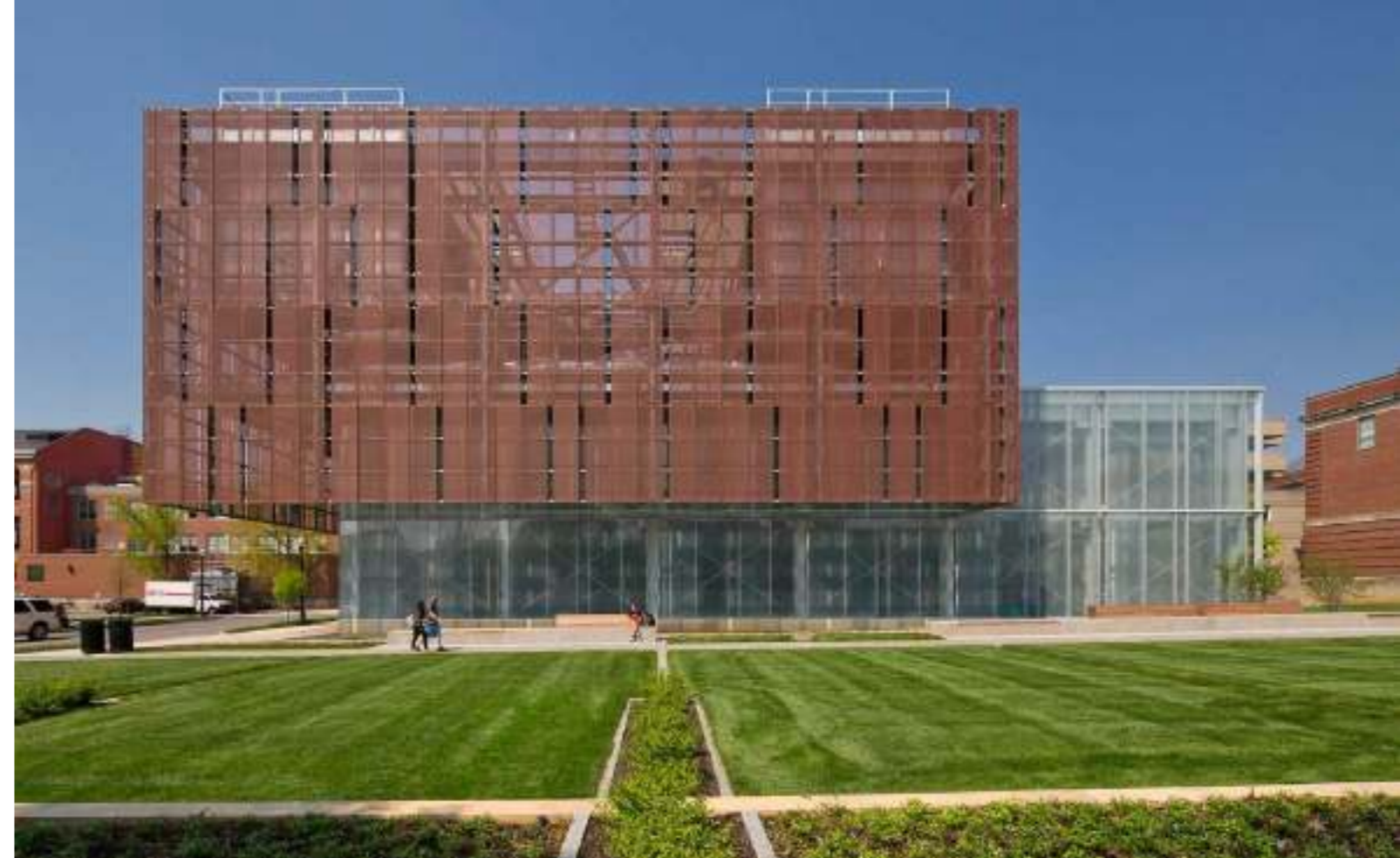
Fig. 1. Leers Weinzapfel Associates, The Ohio State East Regional Chilled Water Plant Columbus, Ohio, USA, 2015. © Photograph Leers Weinzapfel Associates.
