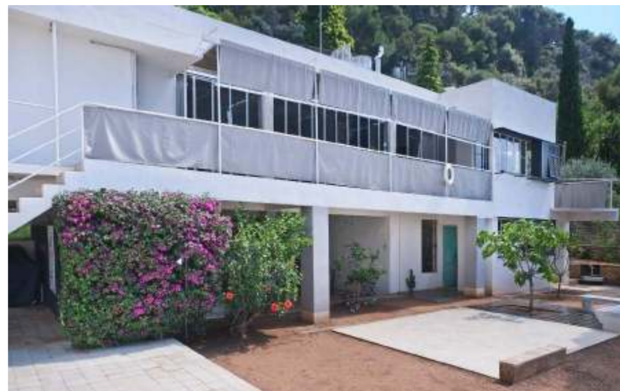
Fig. 1. Eileen Gray's House E-1027 (photo Andrea Furlan, 2018). Courtesy by Association Cap Moderne.
