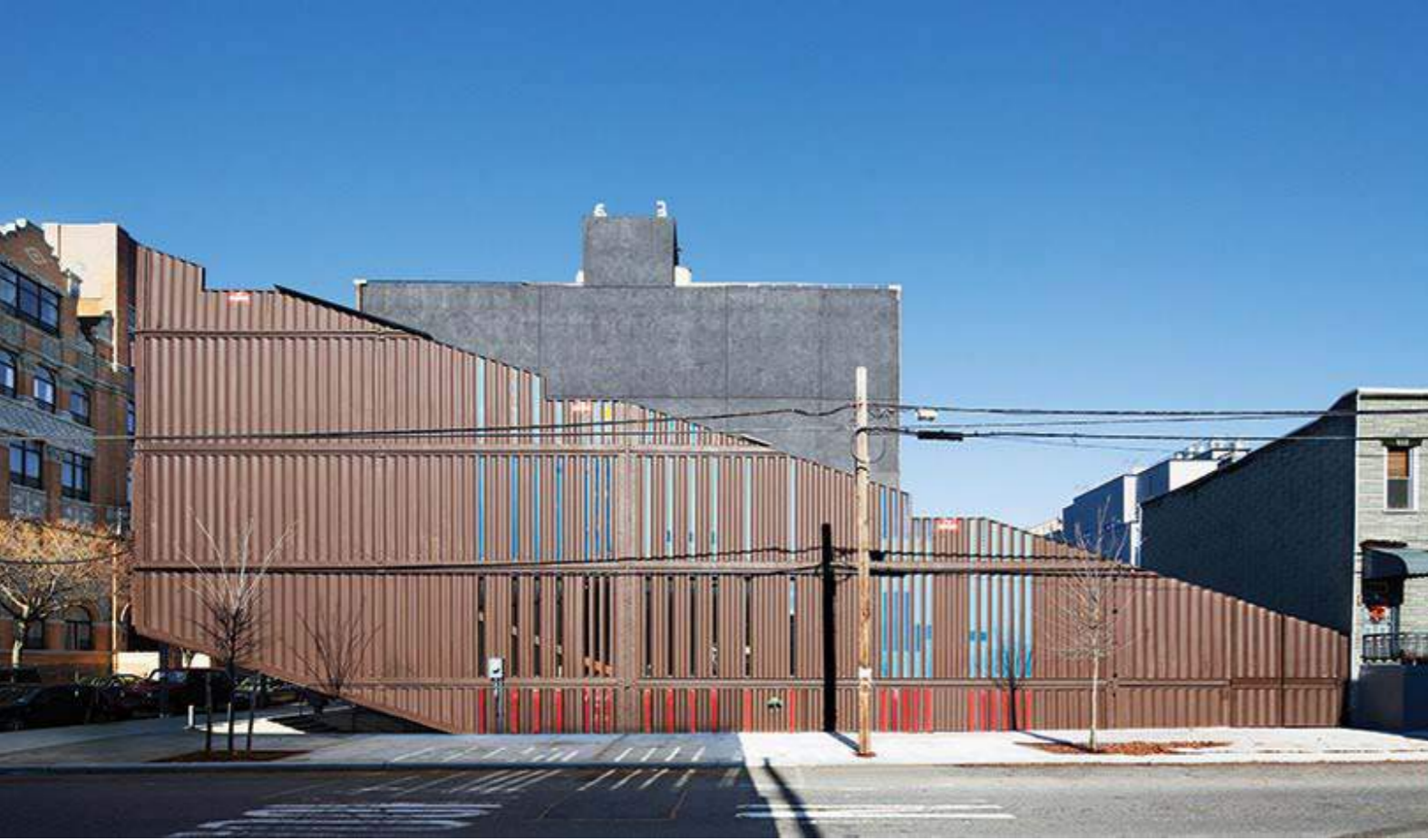
Fig. 1. LOT-EK's Carroll House single-family residence in Greenpoint, New York City, 2012-16, revealing facades made up of recycled shipping container reversed segments resembling Casa Malaparte. Photo: Danny Bright. Source: http://www.lot-ek.com/filter/residential/CARROLL-HOUSE .
