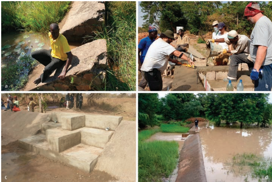
Figure 7. The rebuilding process in Kofeba: (a) the old barrage ; (b) the building phase; (c) the wall complete; (d) the barrage working phase (Source: Authors’).
