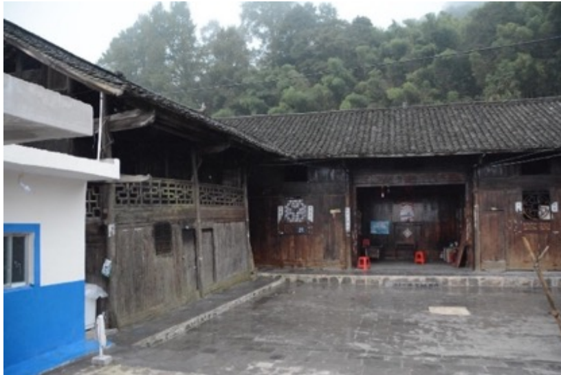
Figure 97: Hu Zhengyong's Dwelling and Courtyard. Source: author's photo.
