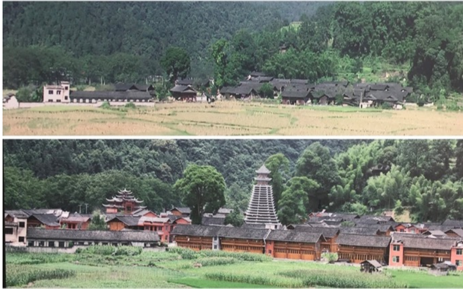
Figure 59: Comparison before and after the implementation of the demolition and reconstruction. Source: Mu Qi (2020). All photos were provided by the Zhaisha village committee during the author's field survey in May 2018.
