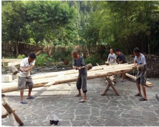
Figure 77: Construction Process Led by the Carpenter Source: provided by Teng Jicheng
