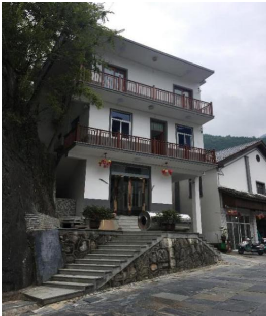
Figure 123: Liyang village, Shangxiang, Zhejiang.. Source: photo by Wang Yipeng, ph.D in Zhejiang University. The author obtained the photo with permit
