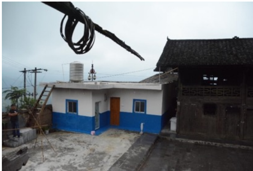
Figure 98: The Plastered Facade of the Toilet of Hu Zhengyong's Dwellings. Source: author's photo
