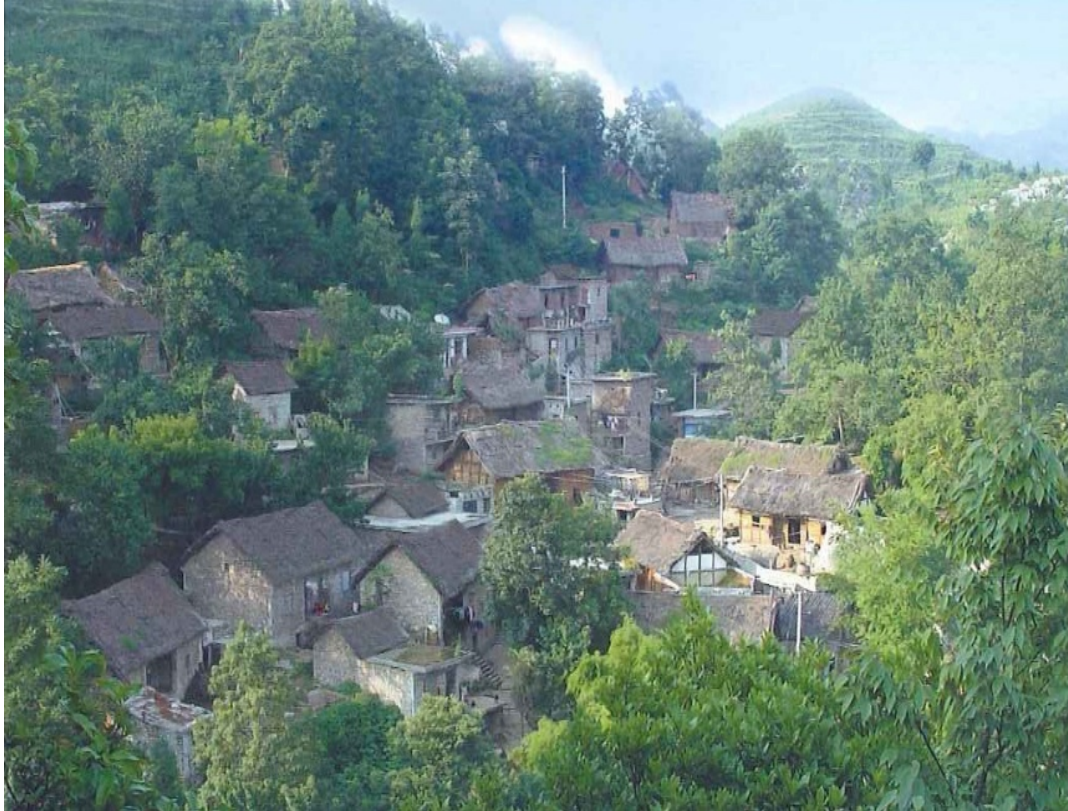
Figure 8: Soga Village in 1998 before the renovation interventions.
