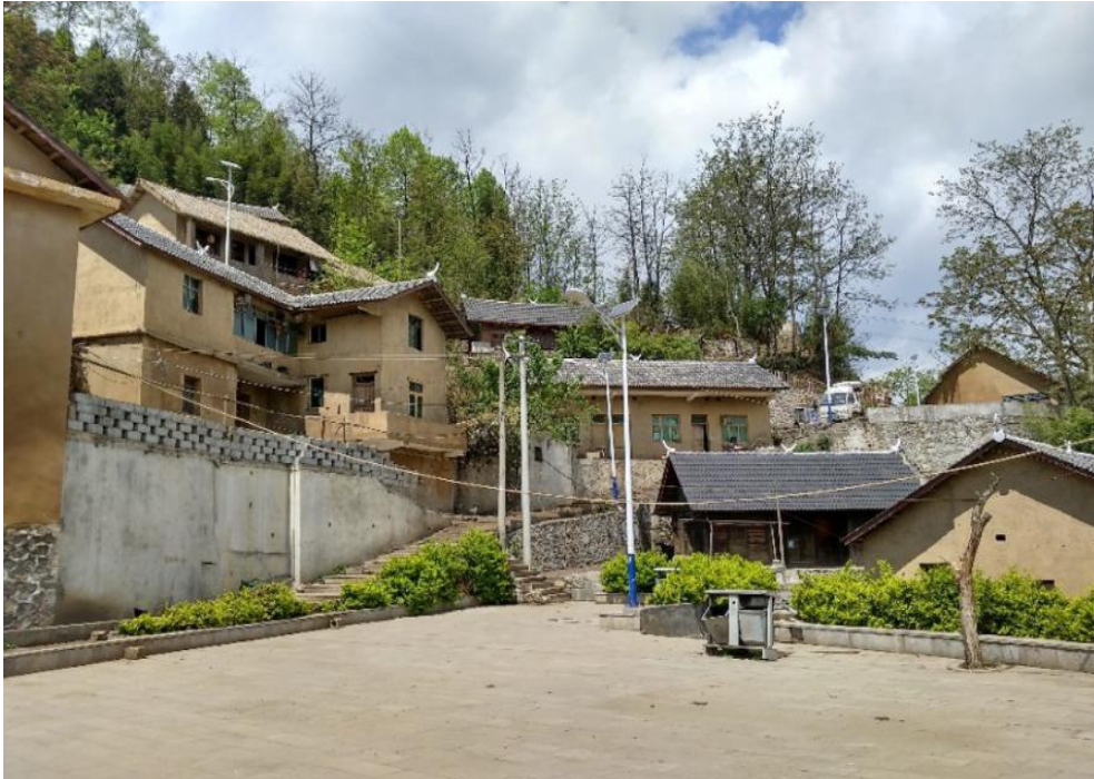
Figure 13: Today's Soga after the renovation interventions. Source: Wu & Huang 2018.
