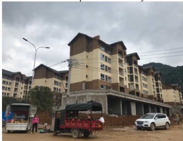
Figure 27: Newly built multi-storey residential buildings in the “new area” to relocate the villagers whose villages have been merged into other administrative villages in the Poverty Alleviation Program in Jiangkou County, Guizhou province. Source: authors' photo taken in May 2018.
