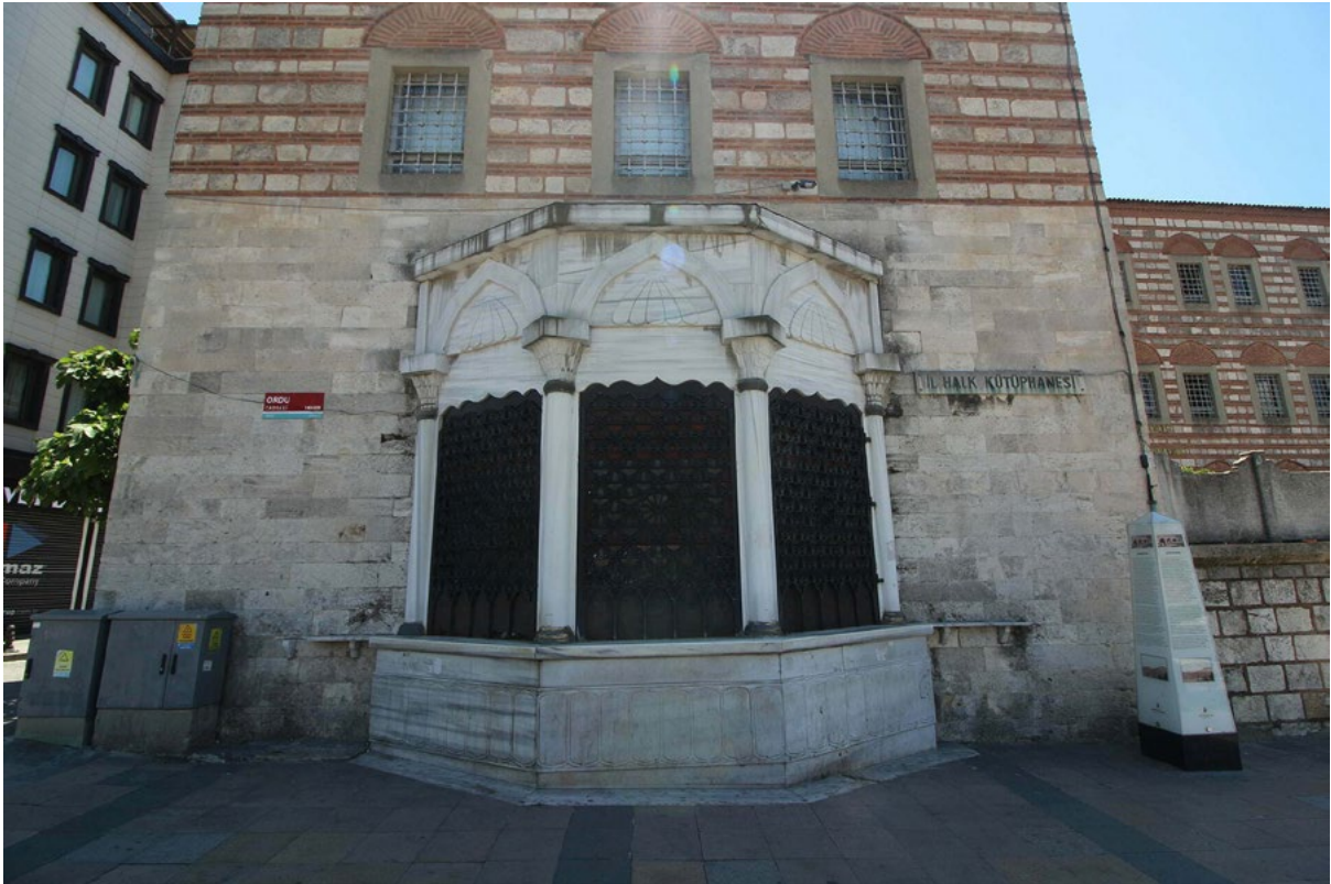
Figure 23. Istanbul. Simkeşhane, reconstruction of the fountain (©Ali Osman Dilekoğlu, https://kulturenvanteri.com/wp-content/uploads/1-289.jpg , access June 29 th 2021).
