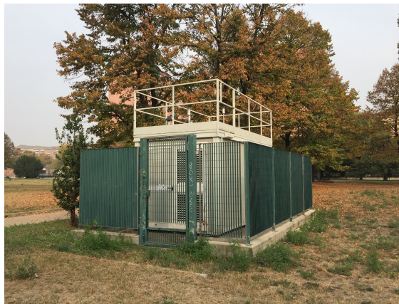
Figure 2.1: The ARPA Rubino monitoring station.
