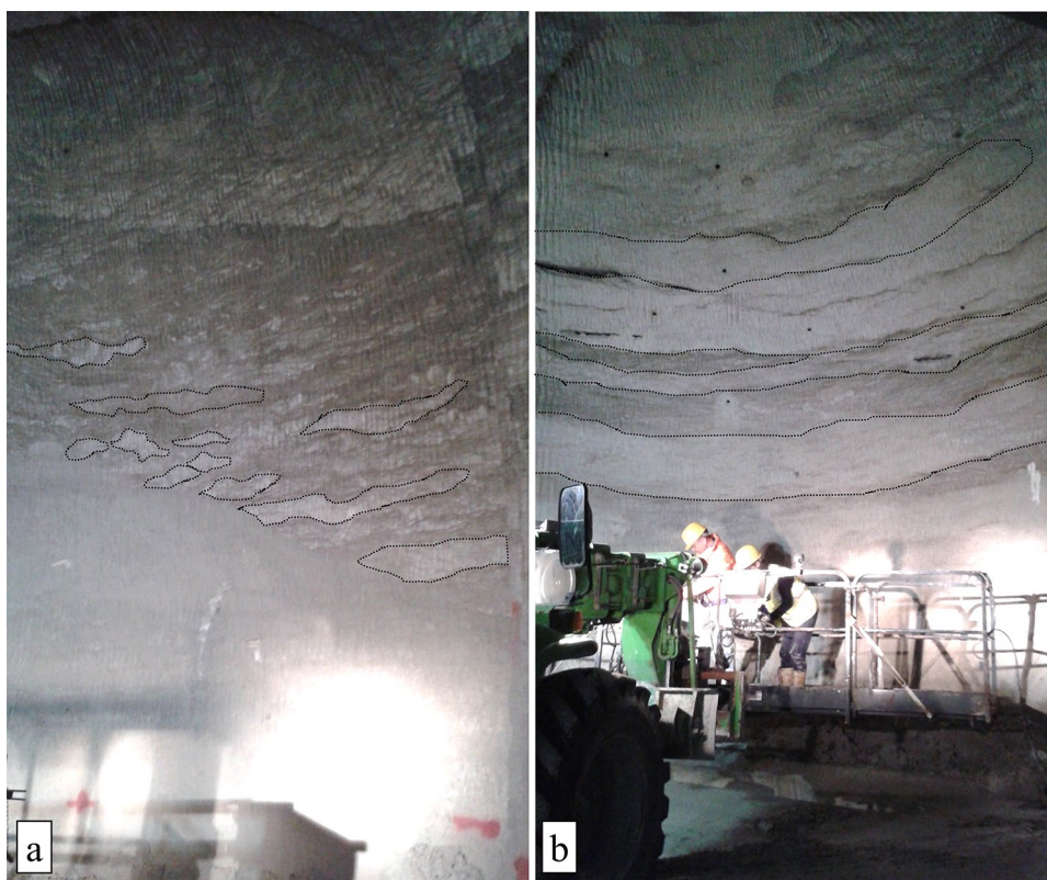
Fig. 27 Excavation faces in underground tunnels in branching selenite gypsum with different macro-textural features. a Small gypsum nodules in a predominant fine matrix. b Big coarse gypsum branches with lower concentration of finer matrix
