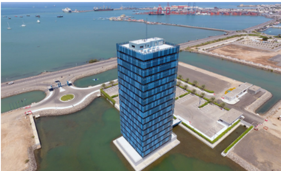
Figure 67: Mezz Group Tower Source: Mezzgroup.Net
