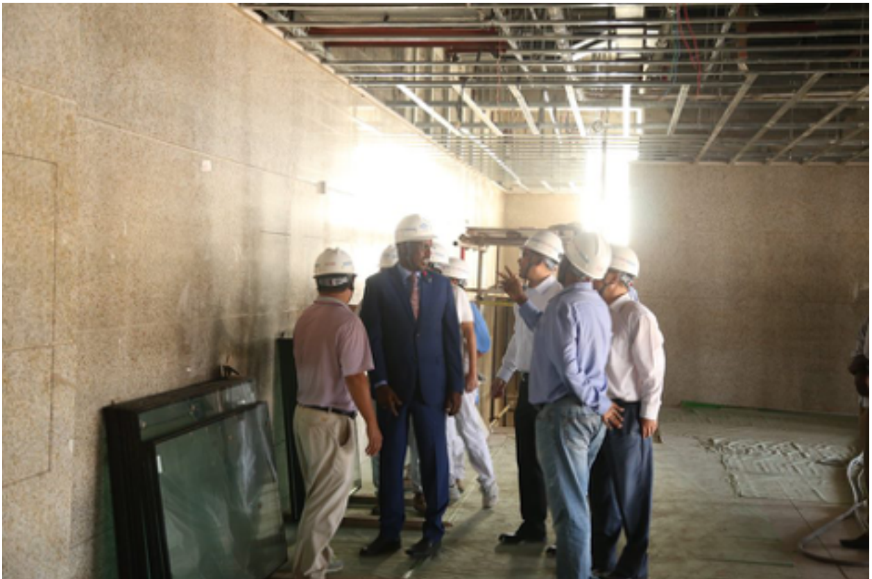
Figure 76: Construction site visit by Minister of Culture Djibouti. Source skyscrapercity.com
