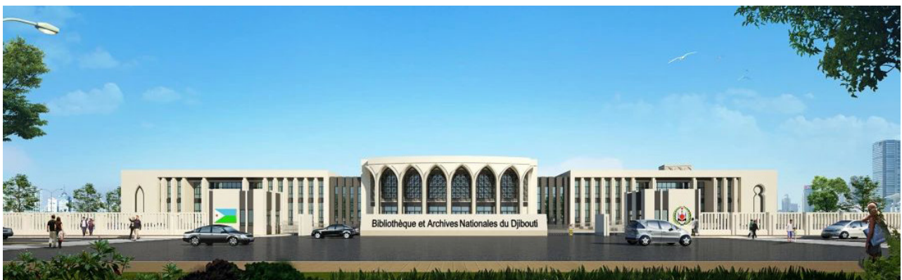
Figure 72: The use of various islamic arches, louvers etc. in China-Djibouti National Library. Source skyscrapercity.com
