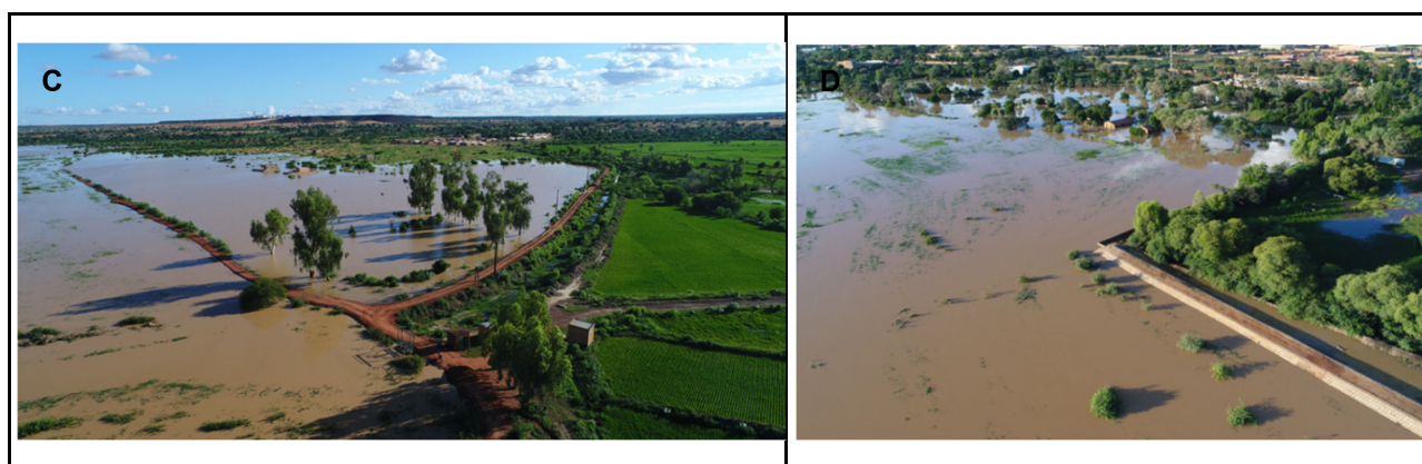
Figure 7. The Niamey levees during the 2019 and 2020 flood events: (A)(top-left) the bridges levee (sector B) raise with sandbags on 18/8/20 ( h = 651 cm), (B)(top-right) the levee break in Lamordé (Sector A) on 6/9/20 ( h = 679 cm), (C)(bottom-left) aerial view of Kirkissoie levee on 30/8/19 ( h = 619 cm), (D)(bottom-right) aerial view of Saga levee on 30/8/19 ( h = 619 cm).
