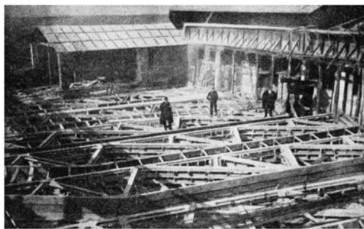
Figure 1. On-site prefabrication of the reinforced concrete truss girders within reusable wooden formwork (Santarella 1931: 346).
