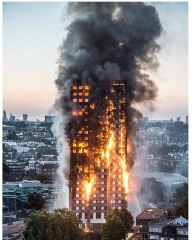
Grenfell Tower fire, 2017, 72 victims
