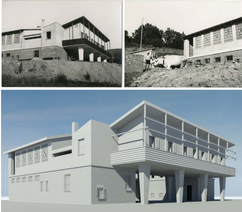
Fig. 10. Comparison of archival photos and clay render of the reconstructive model. (Photos: Archivi BCA. Fondo Aldo Morbelli, BIM Modelling: F. Natta).
