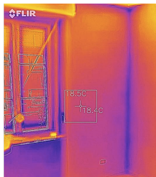
Fig. 3. Thermography of an external wall after the nanotechnology-based insulation.
