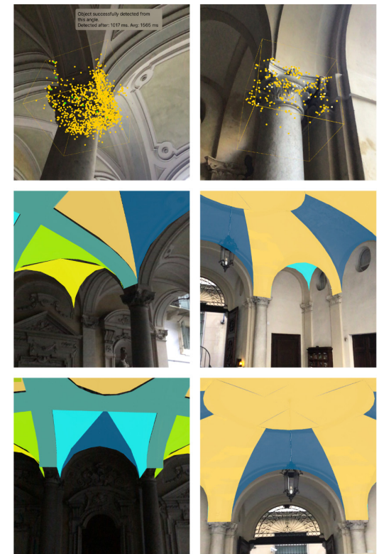
Fig. 6 - Scanning of target object features and superimposition of 3D models in the palaces d'Arcour and Coardi di Carpenetto. Illustration by V. Palma.
