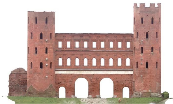
Figure 6. Orthomosaic of the north elevation of the Porta Palatina produced starting from the texturized model
